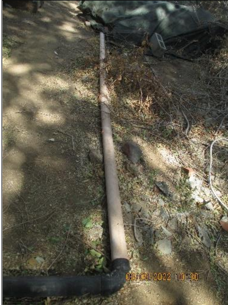
Image 7: Pipeline connected to the pipes pictured in Image 3. Continued under covered debris pile.
