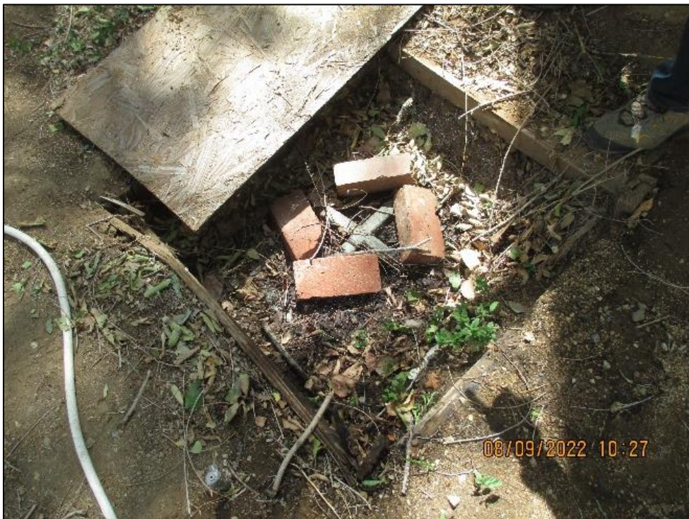
Image 5: West Cesspool cover had red bricks on top. White hose located on the left of the image is connected to potable water faucet.
