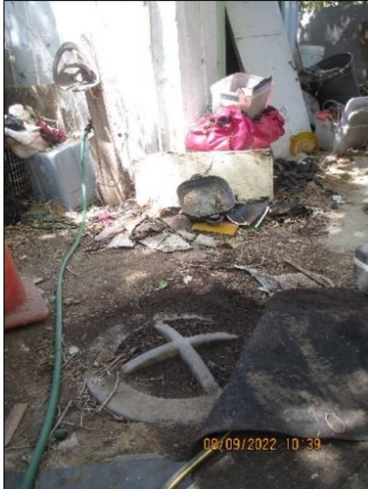
Image 10: East cesspool cover. Green hose and potable water faucet located west of cesspool.
