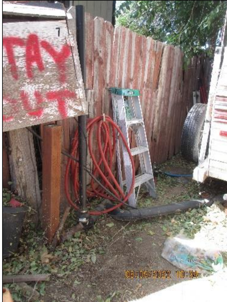
Image 8: Black pipe and vent connected to a mobile home.
